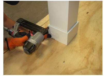
12) Fasten joints on base with pin-nails.
