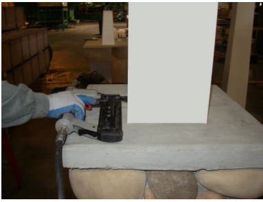
10) Nail column to post ONLY ON THE BOTTOM . Do not attach at center or top (to allow for expansion).
