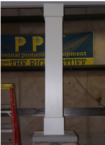
13) The TOP of the shaft should NOT be fastened to the post and there should be at least 1/2" gap to allow expansion (see step 2).
