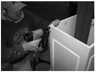
7) Glue and attach final panel. For use as a newel, additional blocking should be added between panels and post (post would be cut off at height of shaft.)
