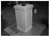
11) Caulk all seams, fill all nail holes, and clean surfaces with cleaner recommended by paint manufacturer. Finish with two coats of acrylic latex paint.
