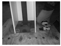
6) Slide the three-panel shaft unit over the blocking, then attach. Apply glue to exposed vertical edges of panels.
