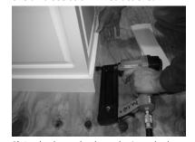
8) Apply glue to backs and mitered edges of base moldings, then assemble to bottom of platform (same as no-taper column bases).
