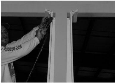
10) Raise 3/4 cap platform section to beam/soffit, center, and attach. There should be 1/4" space for expansion between column and cap platform.
