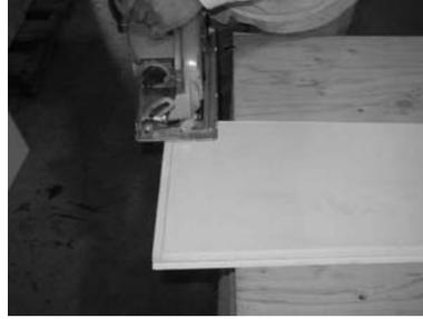
2) Trim shaft pieces to 2 1/4" shorter than opening - 2" for cap/base, 1/4" for expansion (1/4" if not using cap and base - each part is 1" thick.) Always trim from bottom ONLY - top is marked.
