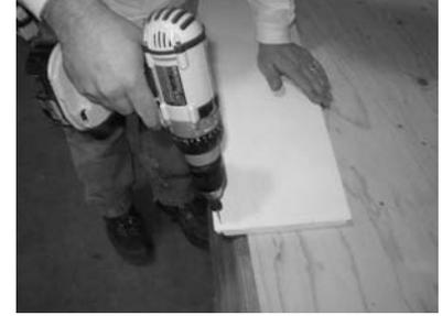
3) If you are going to use screws, pre-drill/countersink all panels. See joint diagram on next page to determine which edge to pre-drill.
