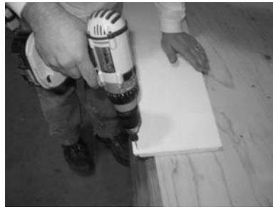
5) If you are going to use screws, pre-drill/countersink all panels. See joint diagram on next page to determine which edge to pre-drill.
