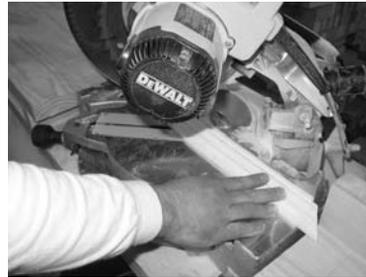
17) Using miter saw, cut base trim pieces to fit around bottom of column
