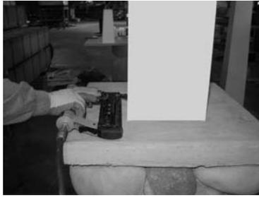
13) Screw or nail column to blocking **ONLY ON THE BOTTOM**. Do not attach at center or top (to allow for expansion.)
