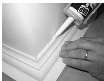
20) Caulk using latex caulking compound to fill any gaps & nail or screw holes.
