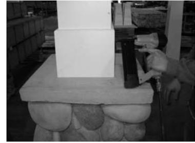
15) Fasten joints on base with screws or nails.
