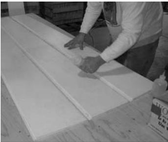
4) Lay 3 panels flat and apply adhesive to center joints. (Polyurethane glue is recommended. Follow manufacturer's instructions.)
