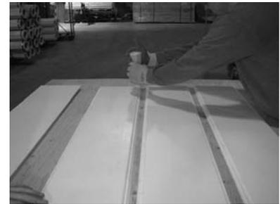
6) Lay 3 panels flat and apply adhesive to center joints. (Polyurethane glue is recommended. Follow manufacturers instructions.)
