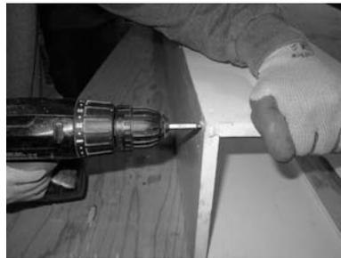
8) If using screws, assemble three panels together using coarse thread galvanized screws (deck screws.)
