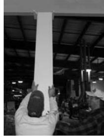
14) Assemble final panel to column using E-Z lock joint
