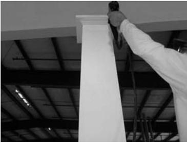
16) Glue ¼ cap piece and slide into place. Pin nail cap moulding to top of column.\*
