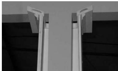
11) Slide 3/4 cap into place on top of column panels.\*
