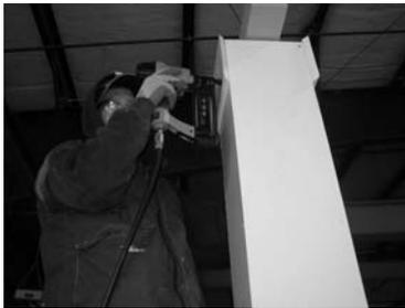
19) Option 2: Leave 1/4" expansion room above cap, and pin-nail the cap to the column. Be sure pin-nails **DO NOT** reach the blocking inside!\*
