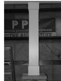
21) Clean surface of column with cleaner recommended by the paint manufacturer. Paint with 2 coats of acrylic latex paint.
