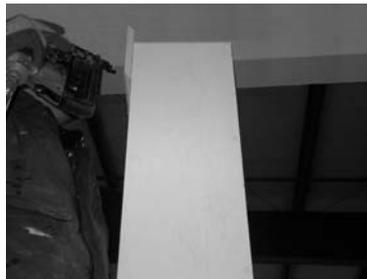
17) There are TWO methods of attaching the cap. First, apply adhesive to mitered ends of cap moulding (7 1/4" tall) and assemble around shaft. Screw or nail joints.
