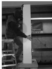
11) Apply adhesive to final panel and attach to shaft using E-Z Lock joints.
