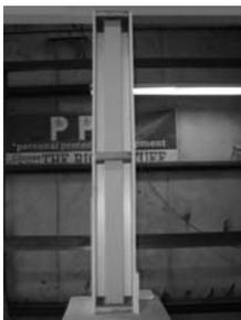
10) Place the partially assembled (3 panels) column around post and blocking.
