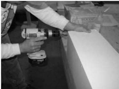
7) If using screws, assemble three panels together using coarse thread galvanized screws (deck screws)
