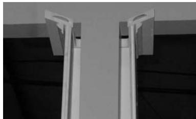
11) Slide  $\frac{3}{4}$  cap into place on top of column panels.\*
