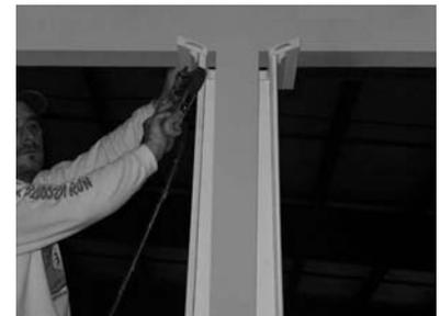
12) Raise cap to beam/soffit, center, and attach. There should be  $\frac{1}{4}$ " between column and cap platform.
