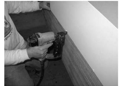
6) If you are not using screws, finish nail three panels together.
