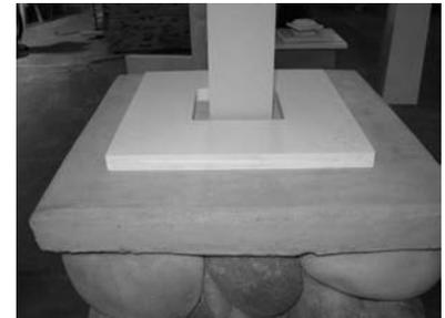
9) Glue  $\frac{1}{4}$  piece of base using biscuits (supplied). Center and attach to floor/pedestal with appropriate fasteners.
