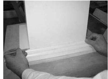
18) Use column shaft to mark cut lines for miters (cut long and work your way shorter for best results)
