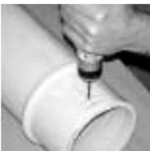
11. Mark and drill clearance holes on the top and bottom of the column to accommodate bolts for the 1 1/2" L-brackets. (L-brackets sold separately.)
