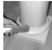
19. Apply caulk to gaps between the cap and base and the column shaft.
