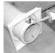
14. Apply construction adhesive to the top and bottom of the column.
