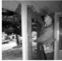
2. Using a jack and post, jack up the beam only enough to remove the sting post, no more than 1/4"
