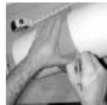
9. Using a piece of cardboard as a guide, draw a line all the way around the column.
