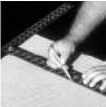
6. Using a square, draw a centerline perpendicular to the outside edge of the platform.
