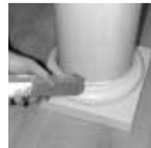
19. Apply caulk to gaps between the cap and base and the column shaft.
