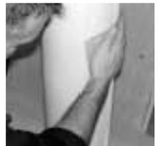
20. Prepare the column for painting by sanding lightly with 120-grit or finer wet/dry sandpaper.
