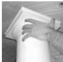
18. Slide the cap up to the beam and push up until secure. Screws may be used to secure the cap to the beam and the base to the platform (When using screws, first drill pilot holes and fill with putty to cover screw heads).
