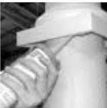
16. Apply construction adhesive to the cap and base.
