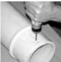
11. Mark and drill clearance holes on the top and bottom of the column to accommodate bolts for the 1" L-brackets (L-brackets sold separately).
