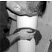
21. Remove dust by wiping the column, cap, and base with soap and water.
