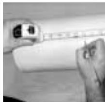
8. Measure from the top of the column to the proper length and make a series of marks around the column shaft.
