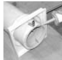
14. Apply construction adhesive to the top and bottom of the column.
