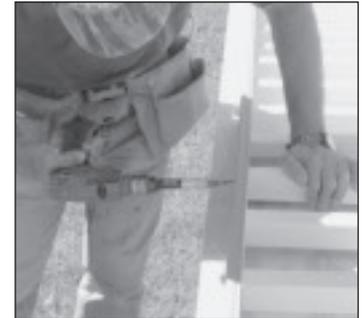
7. Place baluster at center point and screw through bottom PVC rail into baluster. Continue attaching baluster to bottom PVC rail.
