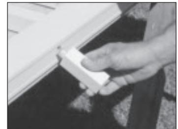
10. If length of rail section is over 4', you will need to install support block. Mark center point of rail section under bottom rail and drill 3/4" hole. Apply non-acetone based construction adhesive on end and insert into hole.
