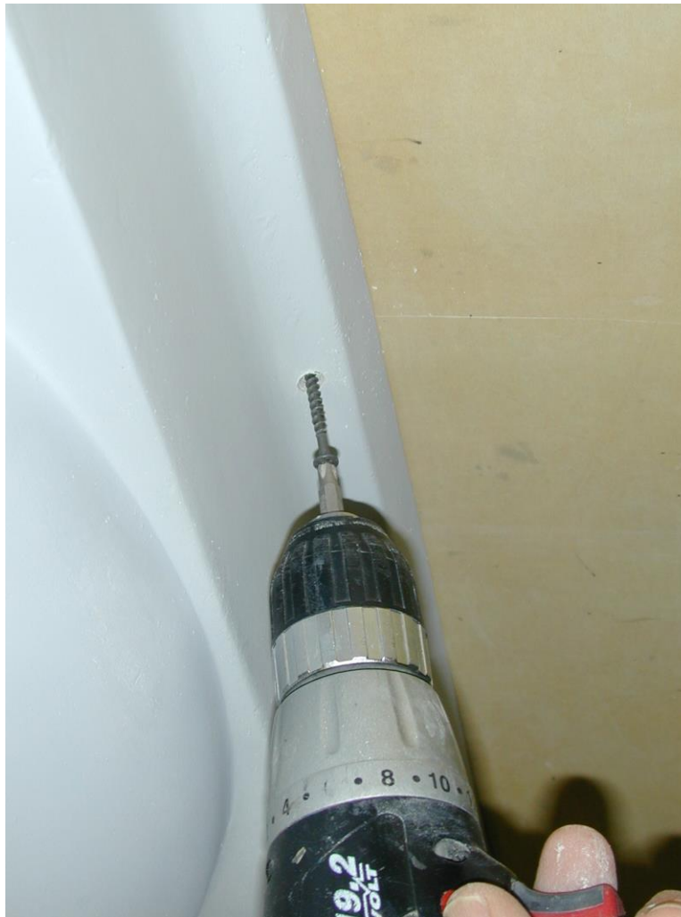
Capital Installation. Pre-drill and countersink before installing screw.
