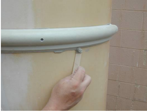
11) Scrape off any excess adhesive.
