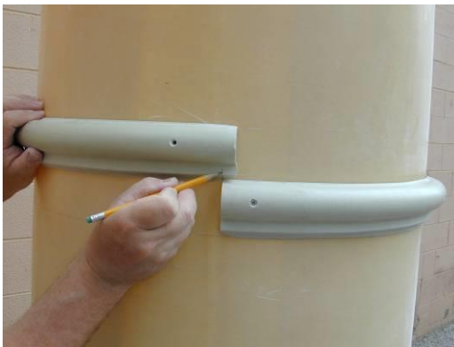
12) Hold the untrimmed neck ring half in position so it can be marked for proper fit.
