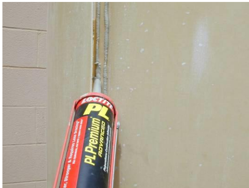
2) After trimming column sections to fit, apply adhesive to joints.
