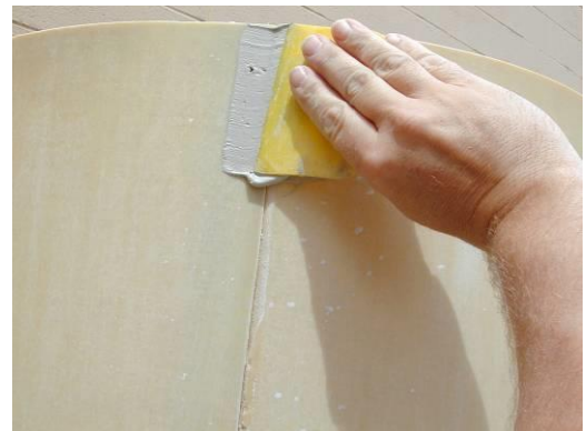
4) Mix body filler (supplied) according to manufacture's instructions and apply to joint. Make joint wide enough to make a smooth radius.
