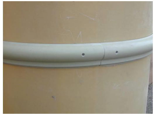
15) Check fit and install the second neck ring half with adhesive and screws.
