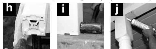
6. Attach plinth to post bottom [h], erect post and drive into position under beam and onto plinth anchoring screw [i]. Drill holes for attaching post to beam, then caulk [j] before using screws to secure.
