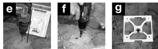
5. Drill platform for plinth anchoring screw [e]. Drive screw to proper depth [f]. Test connection before attaching to post [g]. If using an elevated bracket or aluminum plinth, follow the manufacturers anchoring instructions.
